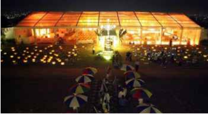
Aluminium "A" Frame Portable Structure - designed, manufactured & erected by FAB INDIA
