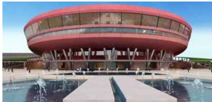
Ongoing Project of I.T.P.O. Convention Centre Building at Pragati Maidan, New Delhi
